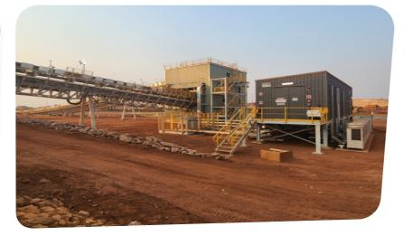
Coastal Electrics installed all LV, HV and communications cabling to the Stock Yard 2 Conveyor system inclusive of all switch room, transformer and field enclosure terminations. The site team completed all phases of testing prior to providing assistance to the client for commissioning.
