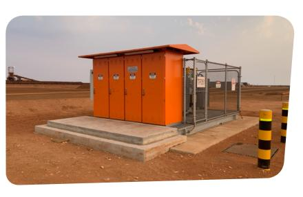
Coastal Electrics Installed 1.5km of 22kV HV cabling and fibre optic cabling from the Concentrate Handling Facility (CHF) to the Concentrate Diversion Pond (CDP), this included the installation and commissioning of one HV transformer, Kiosk Substation, multiple field instruments and pumps.
