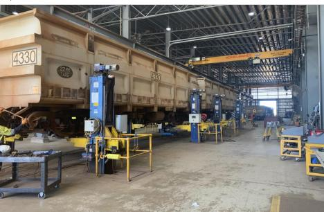
Coastal Electrics provided the installation service & commissioning support for the control systems upgrade on jack systems OP1200 & OP1400. This included the installation of LV cabling, ELV cabling, communications cabling, migration of existing Eurogamma system to Siemens PLC and PLC panel fabrication.
