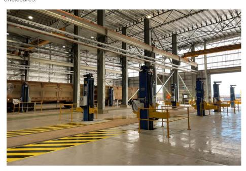
Coastal Electrics completed the E&I package associated with extending the RSM Workshop this included the installation of 2 jack systems, LV cabling, ELV cabling & communications cabling. Along with commissioning support for the OEM & FMG.
